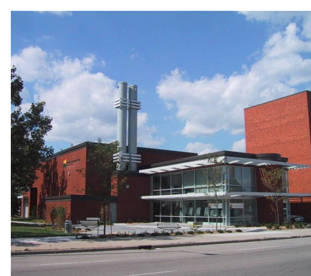
Figure 4 Hamilton Community Energy Centre. (Source: City of Hamilton)
